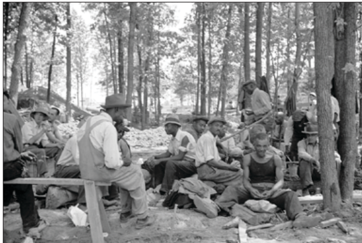
Workers eat lunch at the Greenbelt construction site, July 1936.
