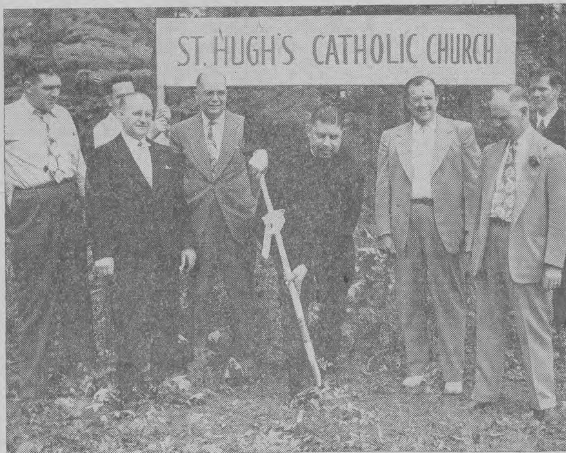
Father Victor J. Dowgiallo, pastor of St. Hugh's Parish, broke ground Sunday for the school and hall to be erected at the Crescent Road site. About 100 Greenbelters were present at the ceremony, including Town Manager Charles T. McDonald and Mayor Thomas Canning, and followed the pastor in removing the traditional shovelful of dirt from the site.
