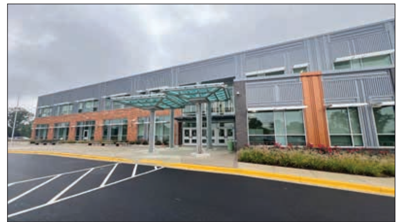
Ellen Ochoa Middle School was designed to meet net-zero energy standards.
