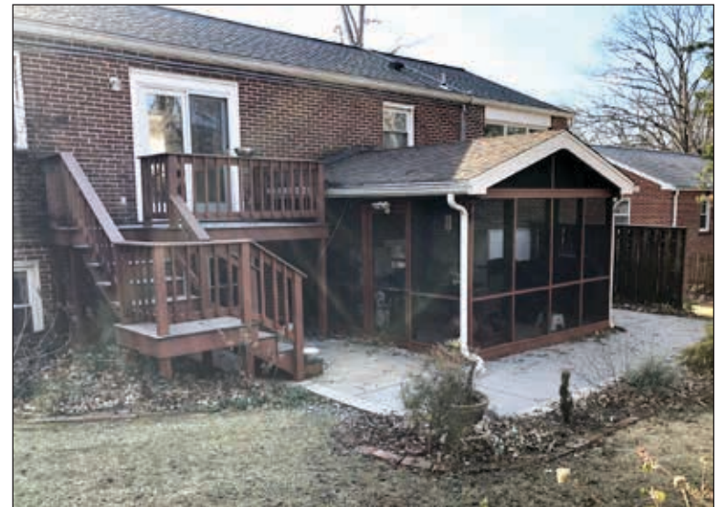
Kash and husband Hank Meyer opened their home's rear wall with a French door for access to the back yard, adding stairs and a screened porch.
