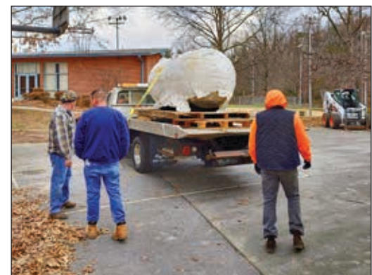
Public Works staff move the new filter into place.
