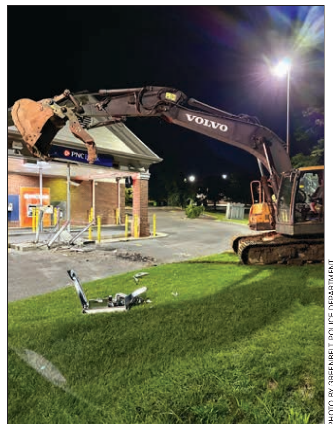
An excavator is left running in front of the PNC Bank. See story, p. 11.
