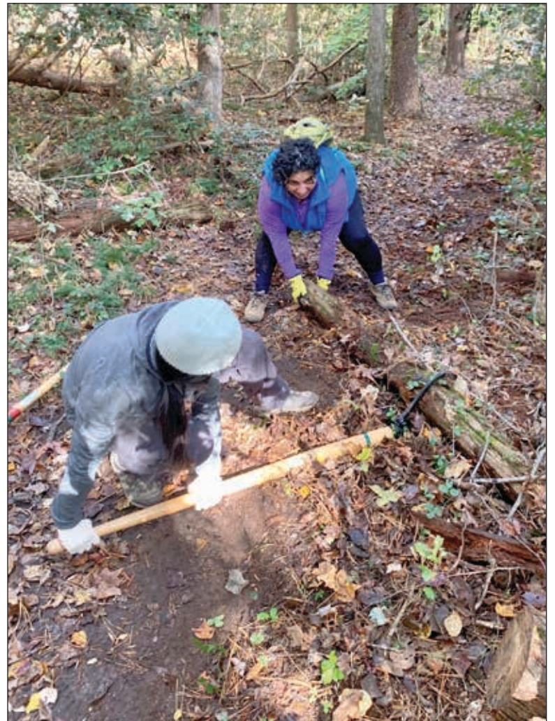
Volunteers Nicole Shyong, left, and Lori Dominick work together using a peavey to move a log.
