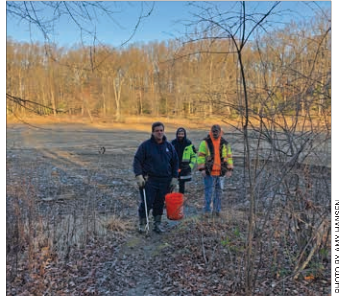
On February 21, Greenbelt public works crew cleans the lake bed of trash washed in via the Lake's feeder streams.
