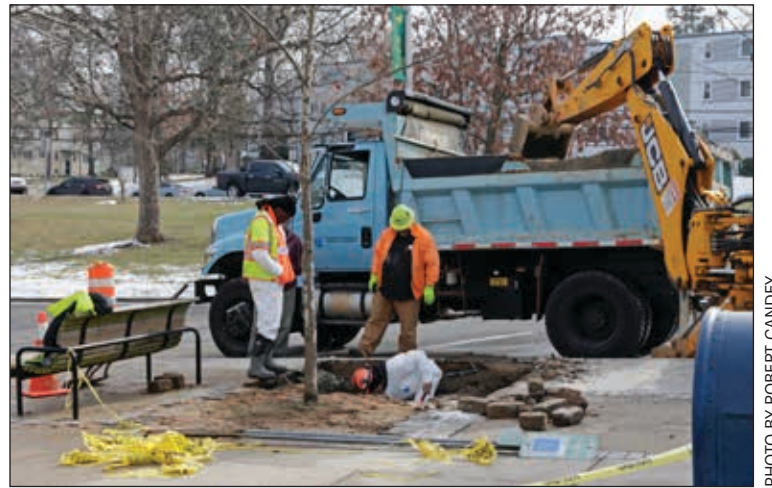
WSSC workers dig down to the pipes under Roosevelt Center.
