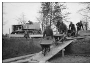
Wheelbarrowing concrete mix from sled to site
