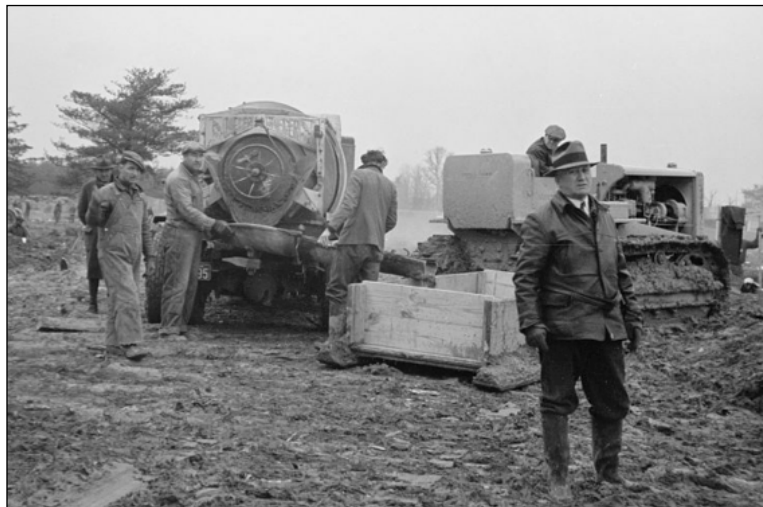
Pouring concrete mix into a wood sled
