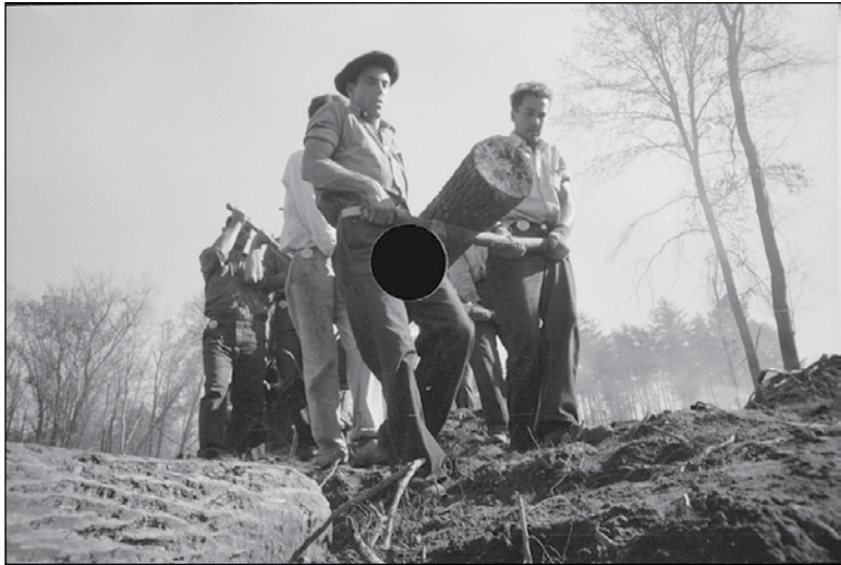
Men hauling a log to build a bridge in Greenbelt
