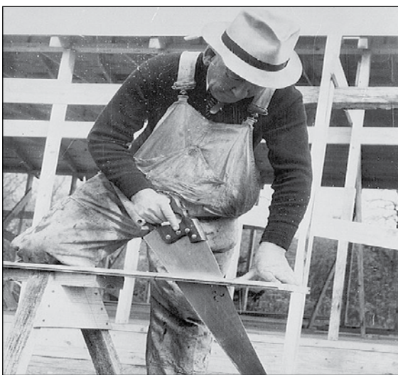
A carpenter working
