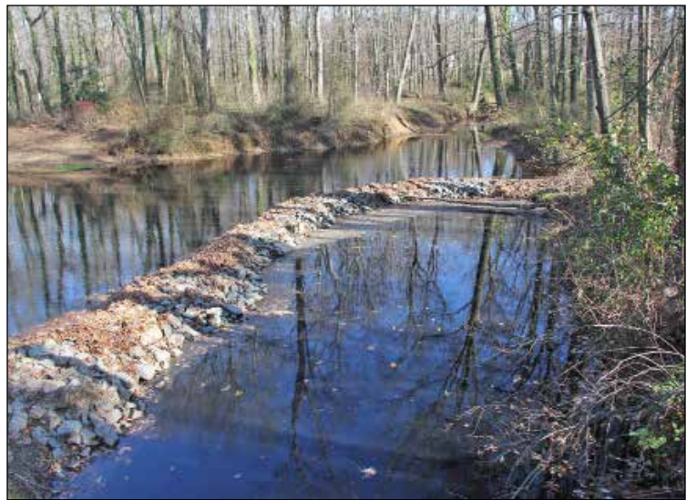
The newly built stone wall slows the water as it moves through the forebay and into Greenbelt Lake.
