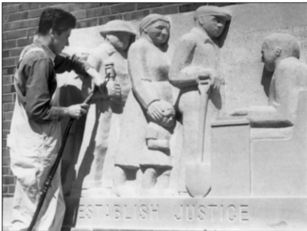
Lenore Thomas Straus works on one of the bas reliefs which decorate the front of the Community Center, formerly Center School, c. 1937.
