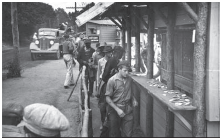
Men arriving at the Greenbelt construction site were required to wear colored buttons designating whether they were skilled, semiskilled or unskilled workers.
