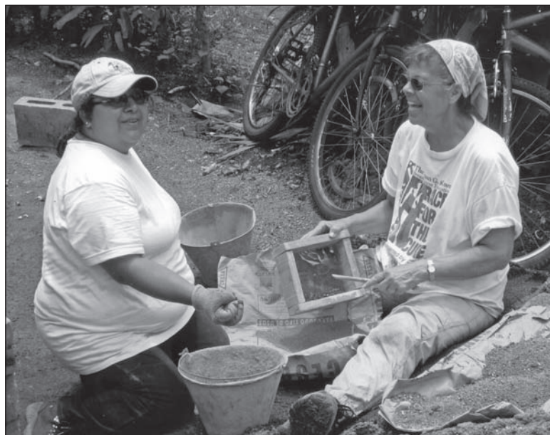
Jean Cook (right) works with Marta Garcia in El Salvador in July 2008. The women are sifting sand which will be used to make cement that will hold windows in place in a house built by Habitat for Humanity.
