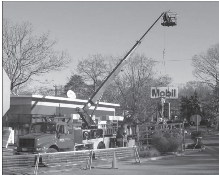
A crane is seen taking down the Mobil sign.
