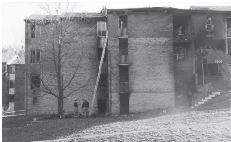
Ladder shows the height of the top floor from ground level.
