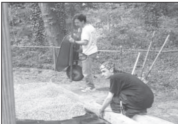
John Norden places wood beam to contain pea gravel.
