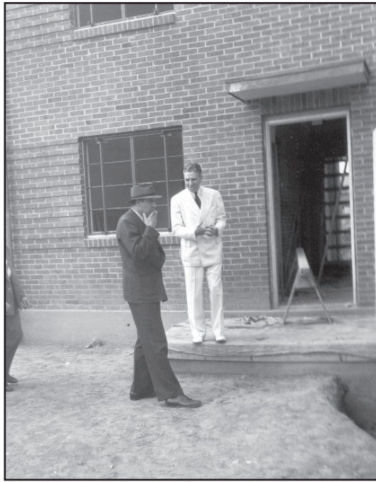
Resettlement Administrator Rexford Tugwell (in white suit) and John Lansill, head of the Suburban Division, inspect a home under construction.
