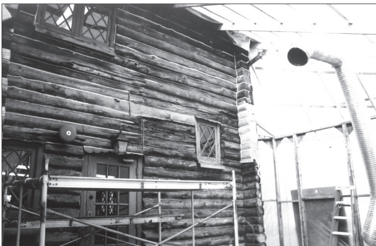
The repair and piecing of logs at the lodge.
