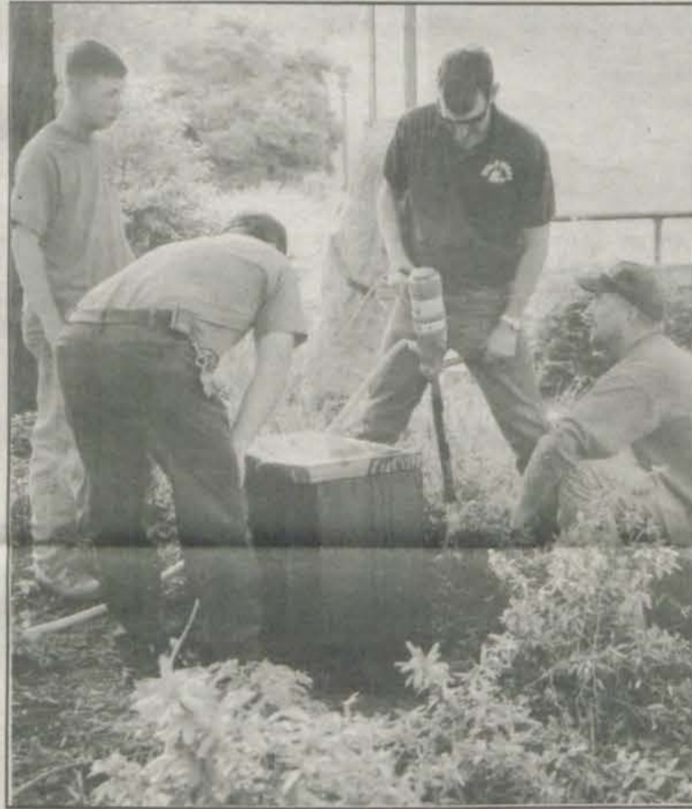
Public works employees constructed the black cement cube that the Lenore Thomas Strauss statue sits on in the new Meditation Garden. A square of black marble covers the rough surface. Here the men prepare to drill two holes for steel pegs that will secure the statue to its base.
