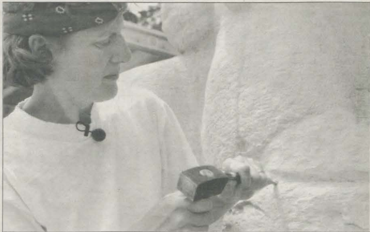
Sharon Koehler shapes the surface of the mortar she used to fill a cleft in the Mother and Child statue, which she is restoring in Roosevelt Mall.
