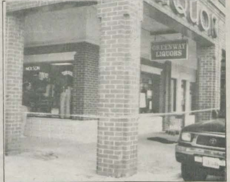
Scene of the crime. A repair man removes jagged pieces of glass left in the broken side window at Greenway Liquors after a deer bounded into the store Monday afternoon.
