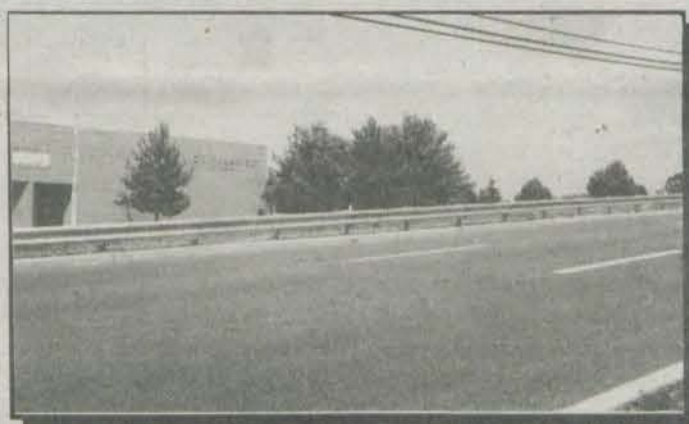
Guardrails were installed along Eleanor Roosevelt High School property.
