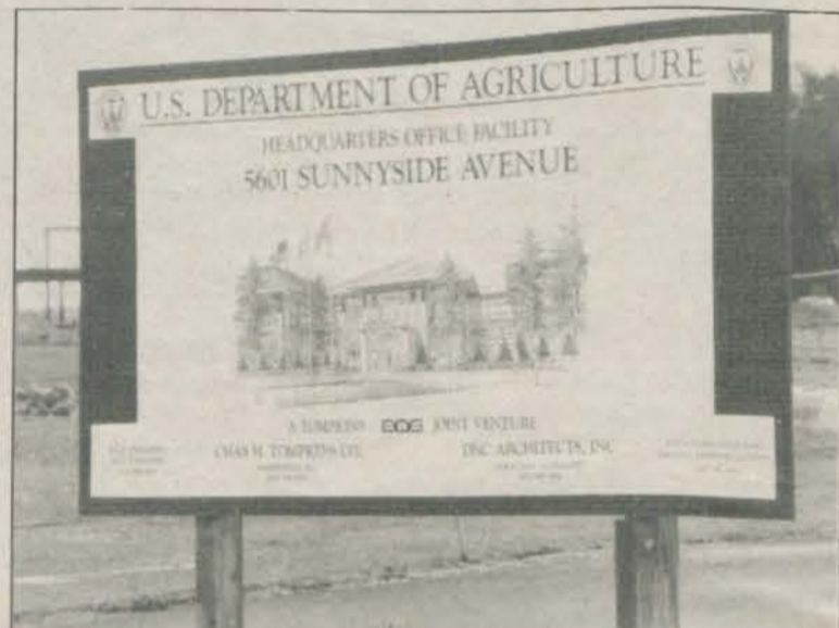
The entrance construction sign for the USDA headquarters facility. -photo by Mary Moien
