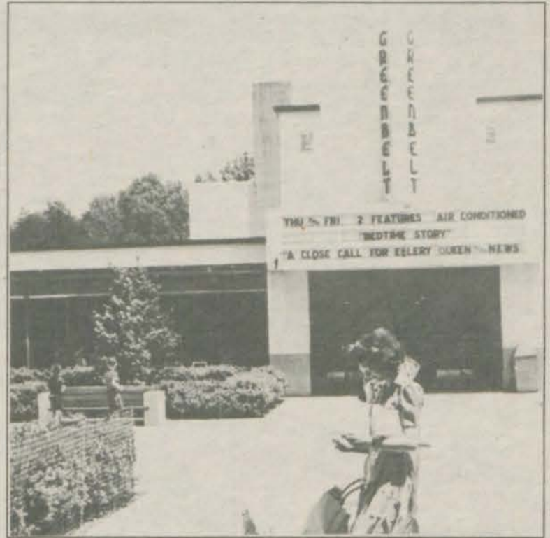
The 1937 design of the Center Mall is partially illustrated in this early photo.
