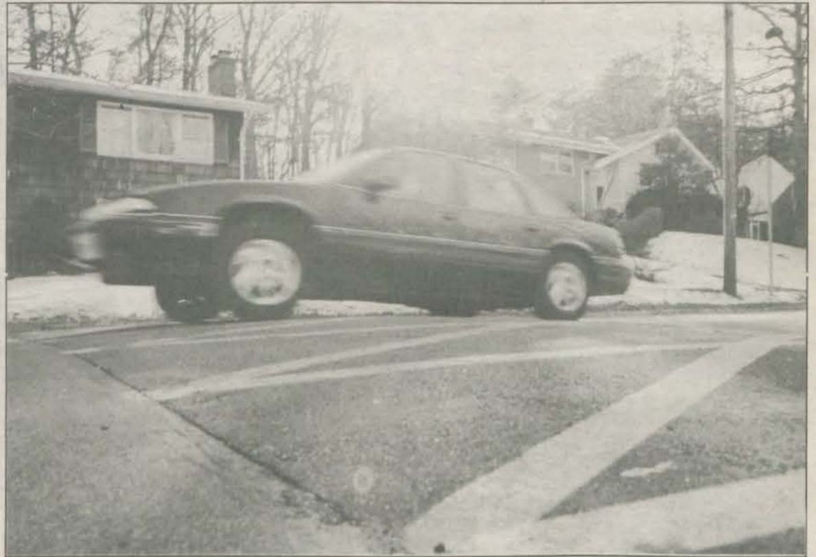
City crews have shaved down and re-stripped the speed humps on Northway. They now can be crossed over at about 15 mph.
