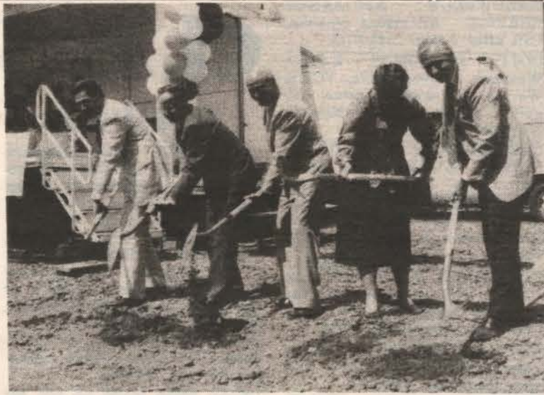
Five members of council dig the indoor pool — Joe Isaacs, Tom White, Mayor Gil Weidenfeld, Toni Bram, and Ed Putens. The ground breaking ceremonies took place Monday after the parade. The new pool should be ready to open by next September. — photo by Nick Pergola
