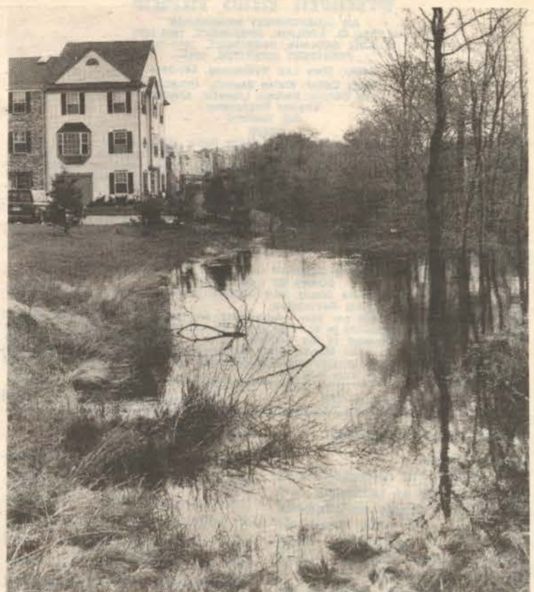
Dammed lake approaches houses in Greenbrook. County bricked up the outflow pipe of the wetlands in Schrom Hills Park. Now water has backed up inundating the wetlands and numerous trees. Photo taken 10 a.m. Tuesday.
