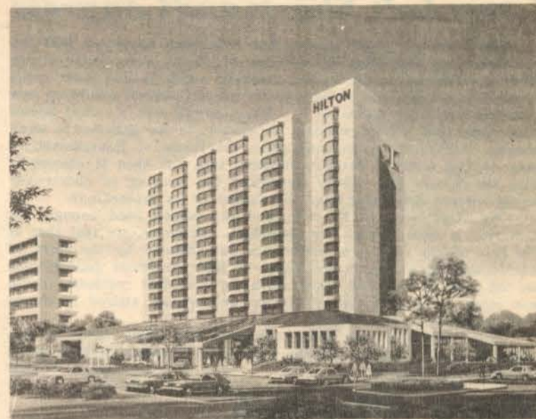
The Hilton consists of a single slim tower for guest rooms resting on a broad base. The material used is predominantly precast concrete so as to harmonize and be compatible with the adjoining office buildings in the Capital Office Park.
