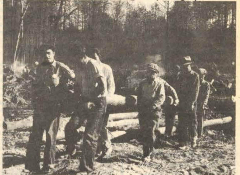
Manpower, not bulldozers, cleared much of the heavy forest covering some areas of the Greenbelt site. Other areas were already farm land.
