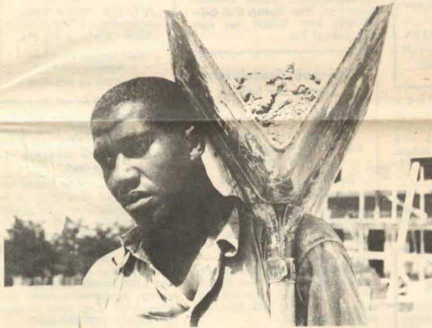
A worker shoulders a load of wet cement which has been mixed on site. All materials and workers came out to the "country" site of Greenbelt by truck and train.
