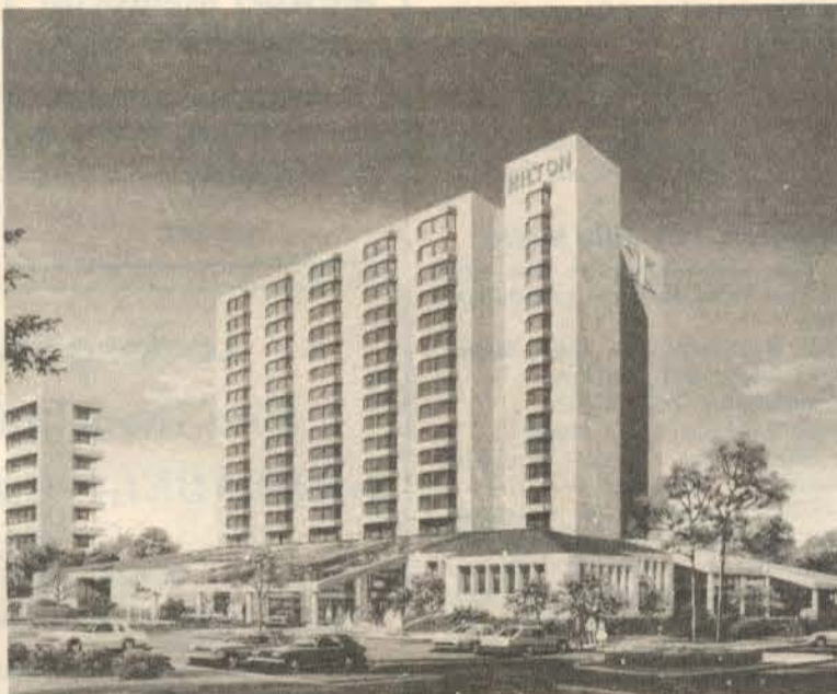
The Hilton consists of a single slim tower for guest rooms resting on a broad base. The material used is predominantly precast concrete so as to harmonize and be compatible with the adjoining office buildings in the Capital Office Park.
