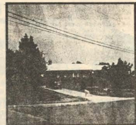
SUNKEN BATHROOM-CAC-2 FIREPLACES -Plus rec room, patio, w/w carpet, washer/dryer, carport and fenced yard. Beautiful setting. All for only a very low price of $69,900. New on market. Call 345-2151.
