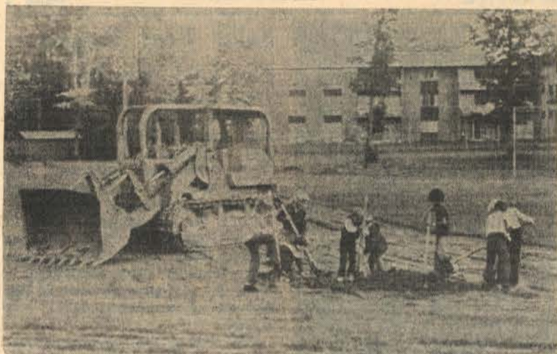
Even the kids got into the act at the groundbreaking. They are helping to dig to speed along construction of the Recreation Center at Springhill Lake.
