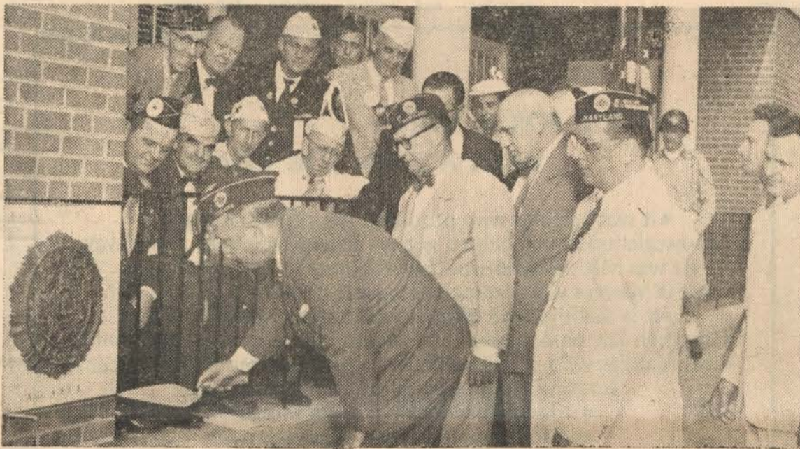
Mayor Frank Lastner (in forefront) overseeing the laying of the cornerstone of the American Legion home on September 2, 1954.
