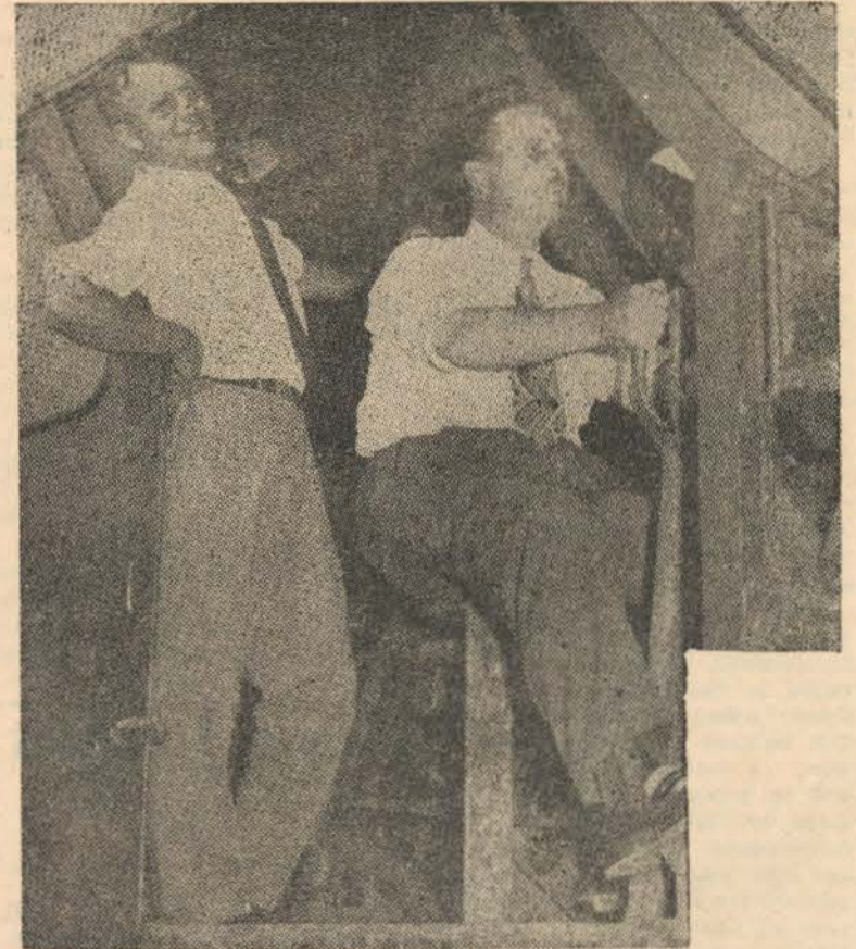
July 1, 1948, GCS President Frank Lastner with back-seat driver Sam Ashelman, Manager of GCS, testing the controls of the crane which was brought in to erect the steelwork for the new co-op supermarket.
