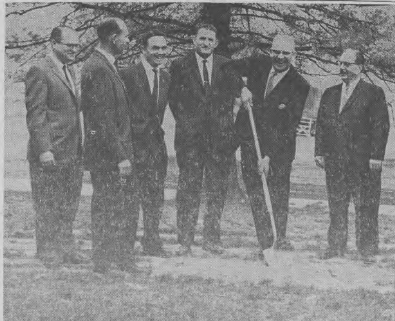
MUNICIPAL GROUNDBREAKING — Digging the first spade of dirt at the April 27 groundbreaking ceremonies of the new municipal building is guest speaker Mayor Joseph F. Lilly of Hyattsville. Admiring his work from left to right are City Manager James K. Giese, Mayor Francis W. White, councilmen William Phillips and Ben Goldfaden, and County Commissioner Frank Lastner.
