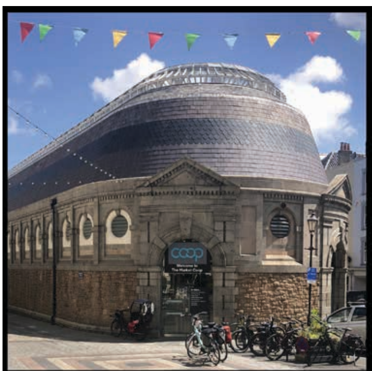
The Co-op building in St. Peter Port, Guernsey, is a lot more fanciful than Greenbelt's.
