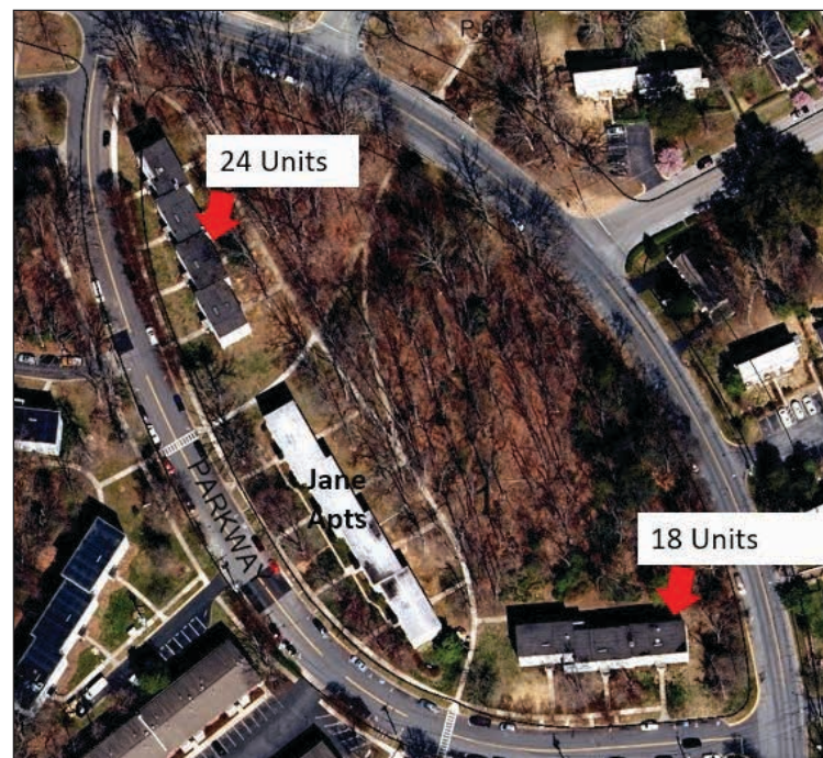
All 42 units at Parkway Gardens are affected by inoperable boiler systems and instead are using problematic window heating units and/or temporary portable units.
