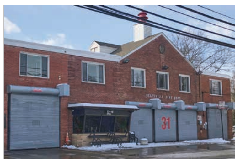
Beltsville Volunteer Fire Department, Station 31, shown on January 11
