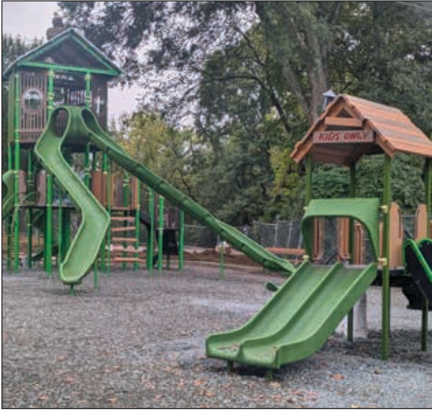
The new Buddy Attick playground nears completion.
