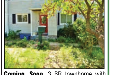
Coming Soon 3 BR townhome with opened kitchen and living room. Cinderblock construction with vinyl siding. One of the largest floorplans in GHI.
