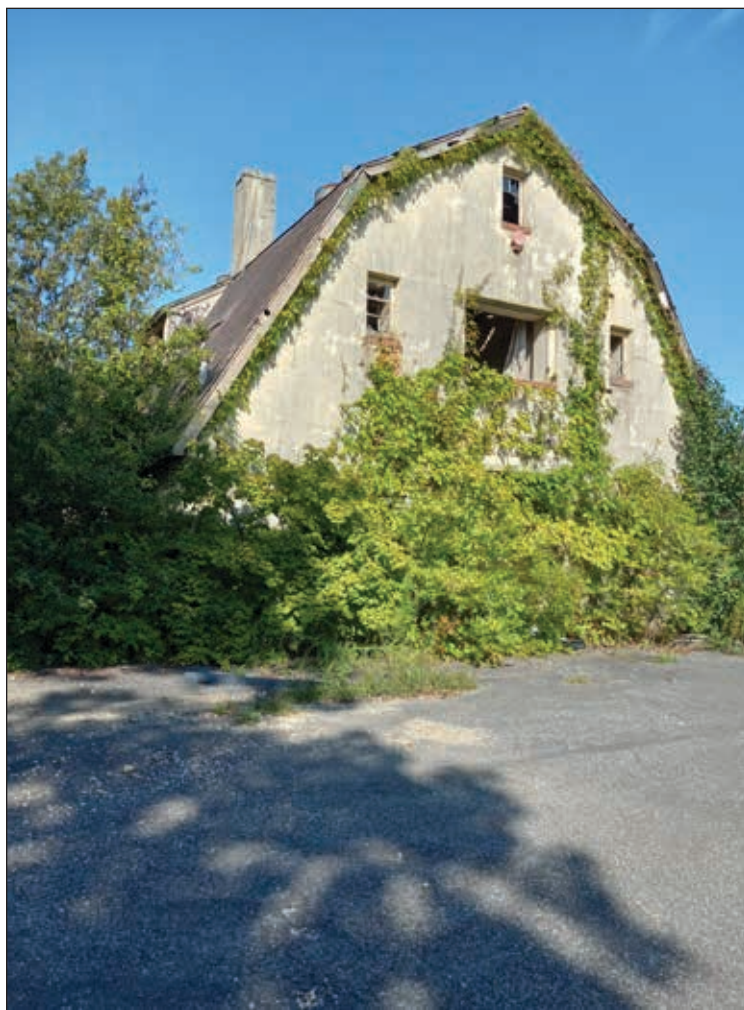
This barn on Zoology Road is on the list of BARC buildings slated for demolition.
