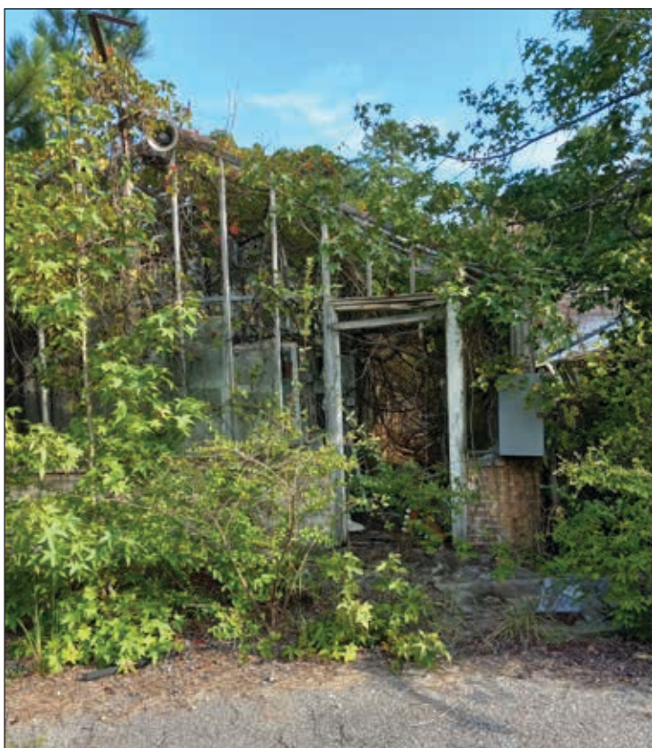
This greenhouse at the end of Entomology Road is slated for demolition.
