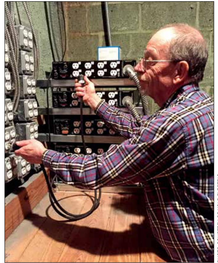
Den Giblin uses the patch panel to select one of the 100 outlets.
