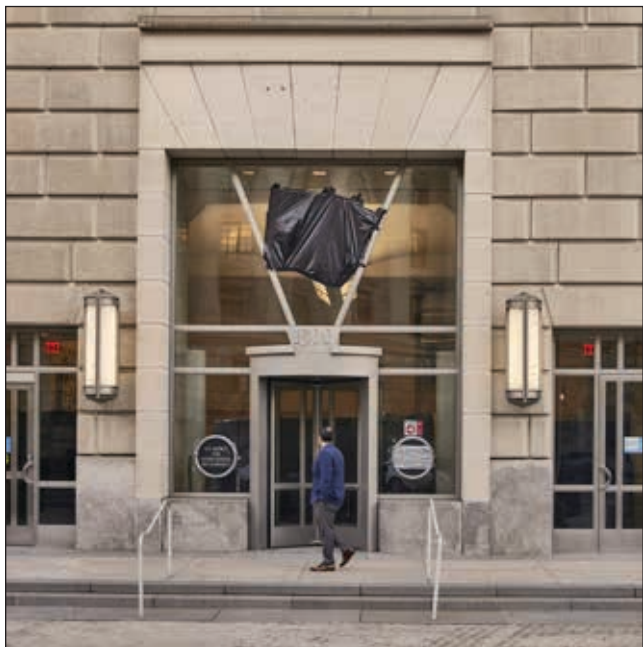
Lettering has been removed from the face of the former USAID headquarters in Washington, D.C., and its signage covered with black tape.
